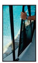
Once fence panels have been installed and tension applied, hang gate by attaching hinges to frame with the self-tapping screws supplied.
